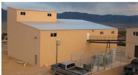
Exterior of the Deer Trail Mill Facility
