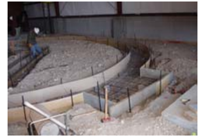
Concrete Footings for Thickener
