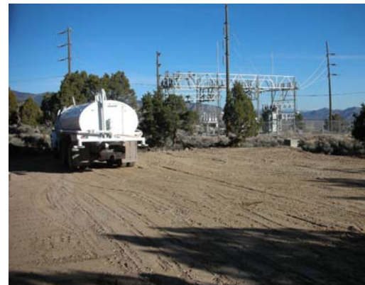
The Substation Site Is Prepared for Groundbreaking and Construction
