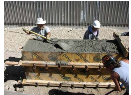
Support Foundation for Catwalk Is Poured
