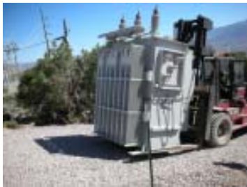
The Main Transformer is Maneuvered Into Place
