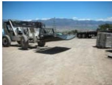
Delivery of Thickener Tank's Rolled Steel Walls
