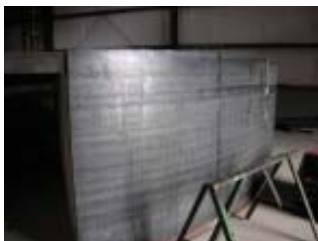
Installation of Rolled Steel Walls for Thickener Tank
