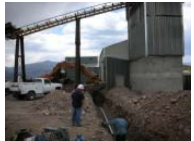
Trench from Upper Water Holding Pond to Mill Facility
