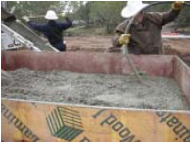
The Cement Pad is Prepared at the Substation Site
