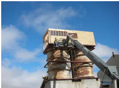
Construction of the upper annex building of the fine ore bins
