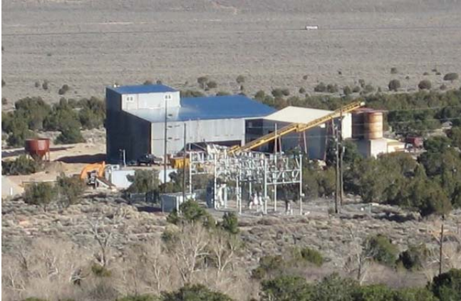
Additional reconstruction work at the mill and processing facility at the Deer Trail Mine has been completed since this site picture was taken in November 2006
