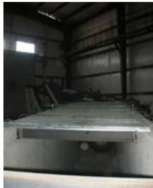
Supports for the upper concrete floor above the conveyor pump slot
