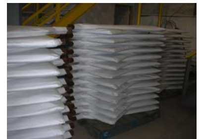
Filter bags installed on the filter sectors
