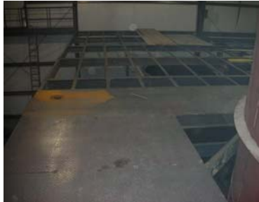
Floor plating for the upper mezzanine in the new mill building
