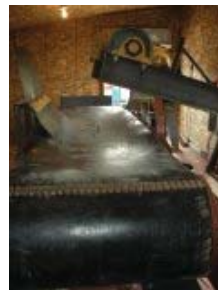
Rubber Belting Installed on Ball Mill Conveyors
