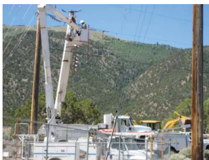
Installation of Power Poles by Rocky Mountain Power Crew
