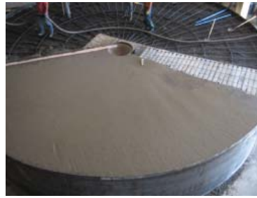
Pouring of the Concrete Thickener Tank Cone
