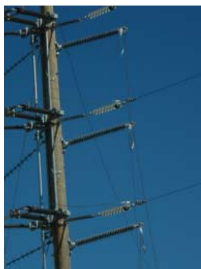
Air Brake Switch Installed on New Power Pole
