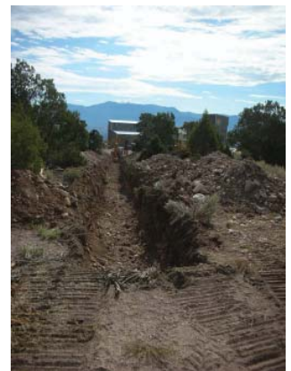
Trench to Secondary Substation
