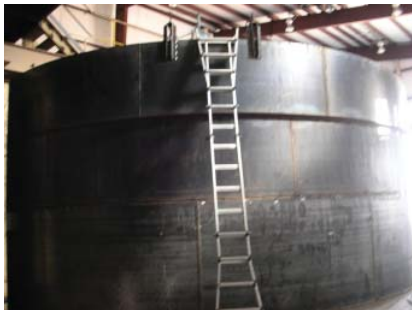
The thickener walls at their final height
