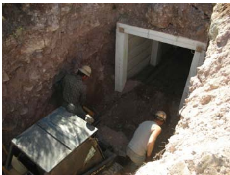
Atlas Mining Begins Underground Mine Maintenance Work
